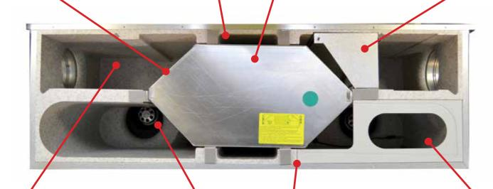
Time-controlled filter change alarm. Easy filter replacement: to open front panels, loosen finger screws. There is plenty of space to replace filters and vacuum the filter space.
