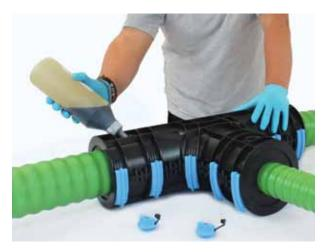
(6) Prepare the two-part PUR foam kit in accordance with the instructions supplied, then pour the mixed foam liquid into the shell through the filling hole.
