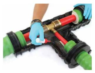
(3) Apply a continuous line of adhesive (4mm wide) to the jointing surface of the lower shell (as pictured).
