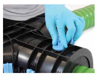
(7) Immediately after pouring foam liquid, seal both openings with the plugs supplied – making a rotary 1/4 clockwise turn.
