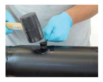
Once poured, both holes need to be blocked with venting plugs down to the first notch. When foam appears in the plugs' vent holes, the plugs can be driven into place with a hammer.
