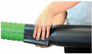
(7) Fit the Heat-Shrinkable Bands Clean the area of the oversleeve and outer casing pipe in the area in which the heat shrink bands will be fitted. Remove the bands from their protective packaging and position them centrally over the overlapping ends of the oversleeve and the outer casing pipe.
