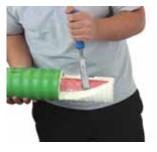
(5) Cut back and remove the insulation along the length (see table for dimension L).
