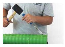
(3) Split the casing pipe with a knife or chisel. Note: Ensure you don't damage the service pipe.
