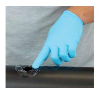
(11) Non-Stick Agent Apply a non-stick agent (such as petroleum jelly or polish) to the areas around the two 25mm holes to prevent excess foam sticking to the oversleeve.
