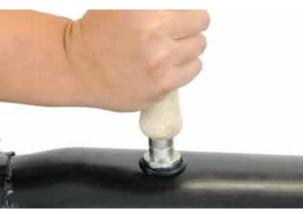
When completed and cooled, the plug should protrude no more than 1-2mm.
