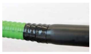
(8) The heat-shrinkable bands can be shrunk down – starting from the oversleeve end. Apply a soft flame from a propane-butane burner. While heating, move the flame in circular movements around the band – taking care not to overheat the area. Repeat this process for the other end of the band – shrinking it down onto the pipe's outer casing – then follow the same steps for the other heat shrink band. Allow both bands to cool before proceeding.
