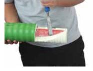
(5) Cut back and remove the insulation along the length (see table for dimensions L).
