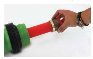
(1) The PEX-LOK compression sleeve can be slid onto the prepared pipe ends. The square end faces the insulation and the chamfered end faces towards the joint.
