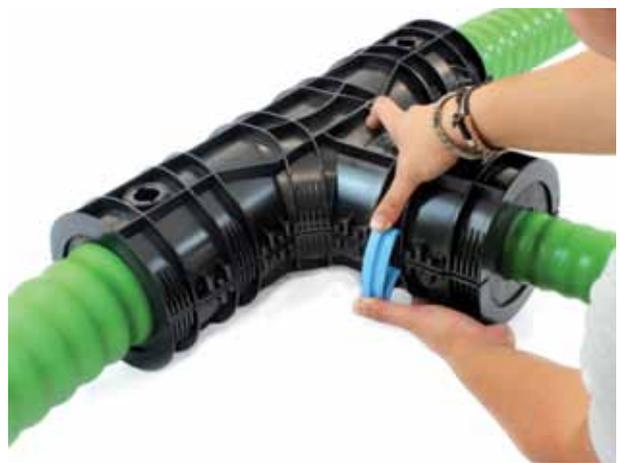
(5) Immediately apply all of the clamps to the locations provided and allow the adhesive to harden for at least 20 minutes.
