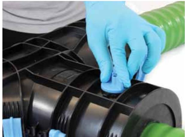
(7) Immediately after pouring foam liquid, seal both openings with the plugs supplied – making a rotary 1/4 clockwise turn.
