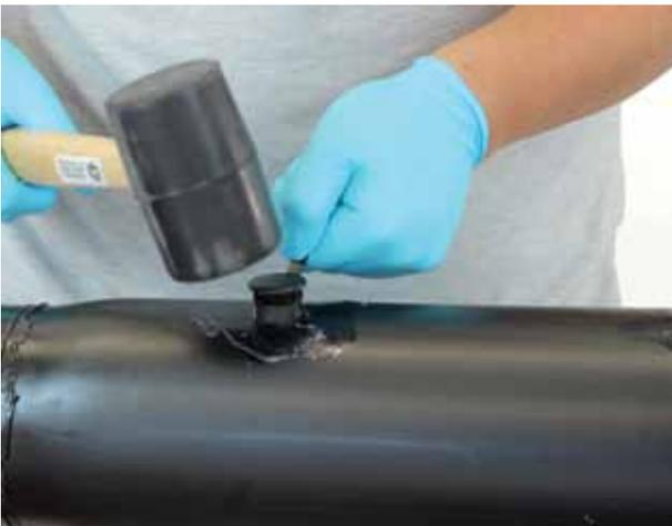
Once poured, both holes need to be blocked with venting plugs down to the first notch. When foam appears in the plugs' vent holes, the plugs can be driven into place with a hammer.
