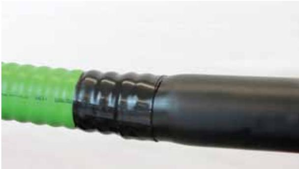
(8) The heat-shrinkable bands can be shrunk down – starting from the oversleeve end. Apply a soft flame from a propane-butane burner. While heating, move the flame in circular movements around the band – taking care not to overheat the area. Repeat this process for the other end of the band – shrinking it down onto the pipe’s outer casing – then follow the same steps for the other heat shrink band. Allow both bands to cool before proceeding.
