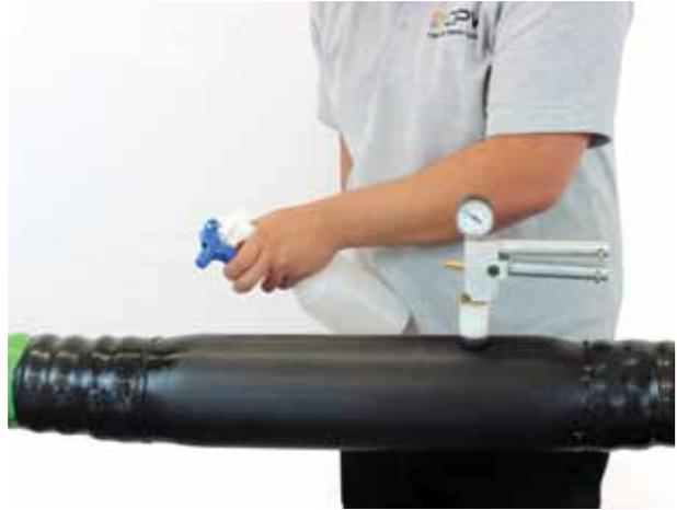
(10) Apply an air pressure test of 0.2 bar for 15 minutes and check for air tightness with soapy water on all joint areas - ensuring there is no drop in pressure. Remove the air test equipment and bore a second 25mm diameter hole approximately 100mm the other side of the centre line on the top of the oversleeve.
