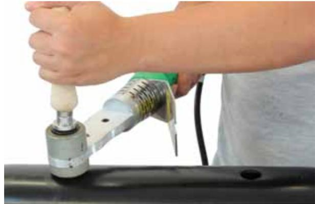
(14) Using a pre-heated electric fusion welding tool, the welded plugs need to be put into the heater, with the male end of the heater placed into the joints filler hole. When heated, the plug can be pressed into place in the hole with hand pressure until there's a visible 2mm bead melt on both the plug and hole. Repeat this process for the second hole.
