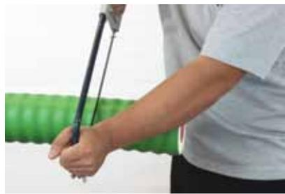
(2) Cut the casing pipe with a saw.
