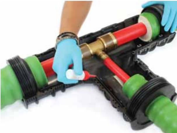
(3) Apply a continuous line of adhesive (4mm wide) to the jointing surface of the lower shell (as pictured).
