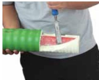
(5) Cut back and remove the insulation along the length (see table for dimensions L).
