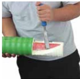
(5) Cut back and remove the insulation along the length (see table for dimension L).
