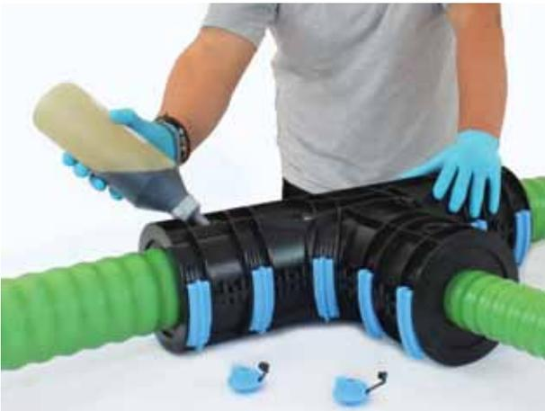
(6) Prepare the two-part PUR foam kit in accordance with the instructions supplied, then pour the mixed foam liquid into the shell through the filling hole.
